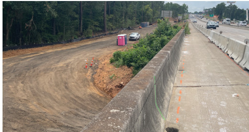
View from the eastbound side of the Saluda River bridge looking west. Installation of access roads and a temporary barrier wall to separate construction traffic from the traveling public is complete.
