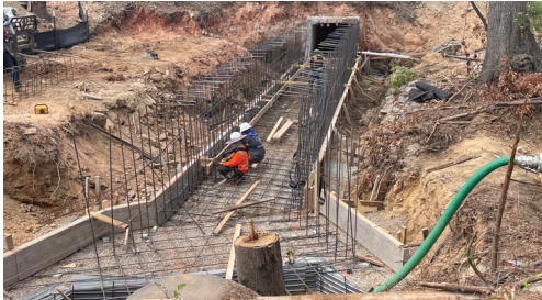
Culvert extension construction along I-20 eastbound.
