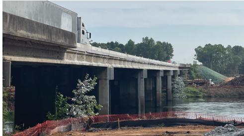
Partial demolition of the I-20 bridge over the Saluda River. The original barrier is gone and a temporary barrier is bolted to the existing bridge deck.
