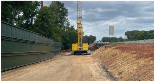
View from the westbound side of the Saluda River bridge looking east toward the river. Mobilization of cranes and barges is underway. These will be used during construction of the new I-20 Saluda River Bridge.
