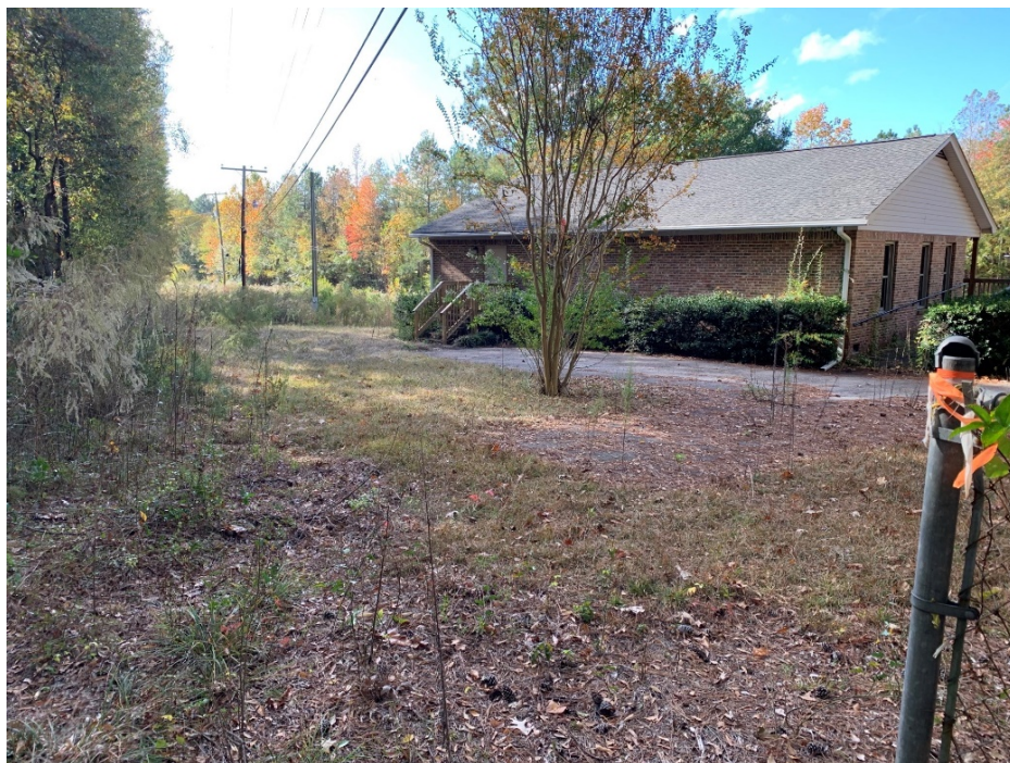
View of Parcel 392, facing south.
