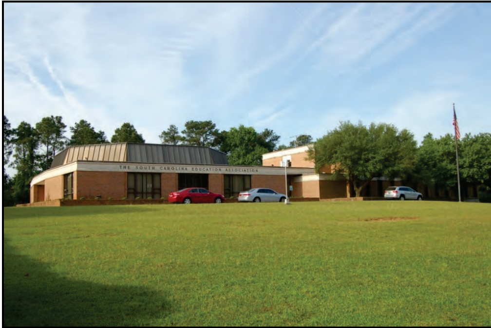
Figure 5.48: Resource 106-0880 (421 Zimalcrest Drive) – View of the facade, facing northeast.
