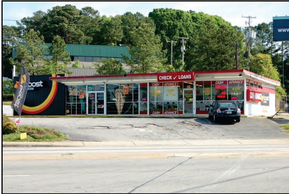
Figure 5.36: Resource 106-6396 (859 Bush River Road) – View of the facade, facing northeast.
