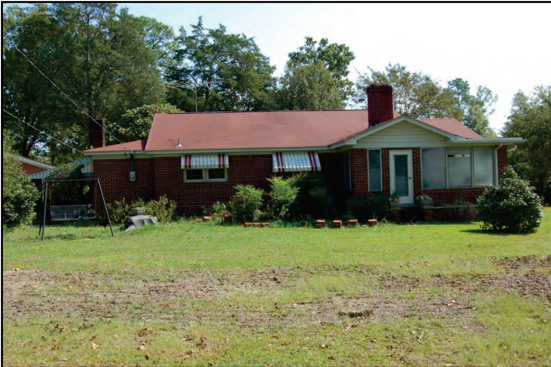
Figure 5.73: Resource 243-6467 (200 Roof Lowman Road) – View of the west side elevation, facing east.
