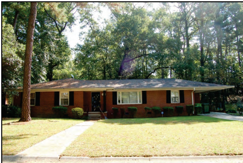
Figure 5.57: Resource 106-6400.02 (Chartwell Subdivision) – Representative view of property within the subdivision located at 124 Chartwell Road, facing southeast.
