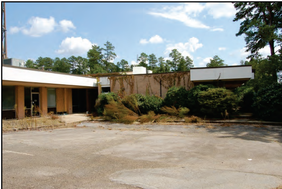
Figure 5.18: Resource 106-6466 (910 Gracern Road) – View of the south side elevation of original portion of resource and façade of later addition, facing east.
