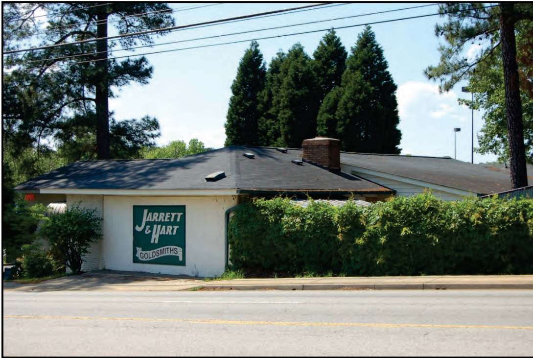
Figure 5.60: Resource 106-6401 (3102 Greenore Drive) – View of the south elevation, facing northwest.
