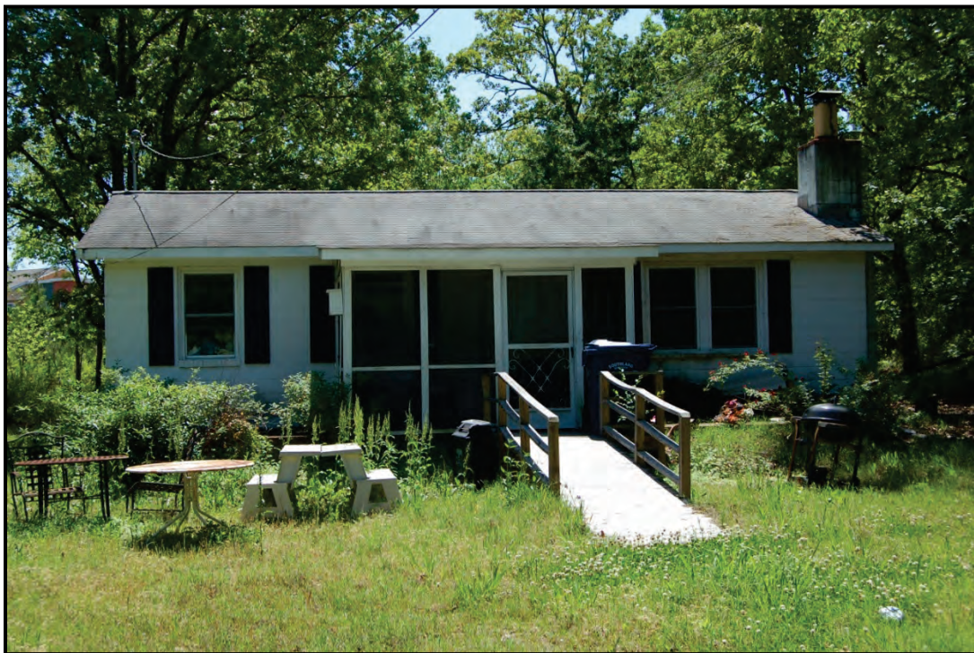
Figure 5.69: Resource 243-6403 (37 Bluebird Trail) – View of the façade, facing southwest.
