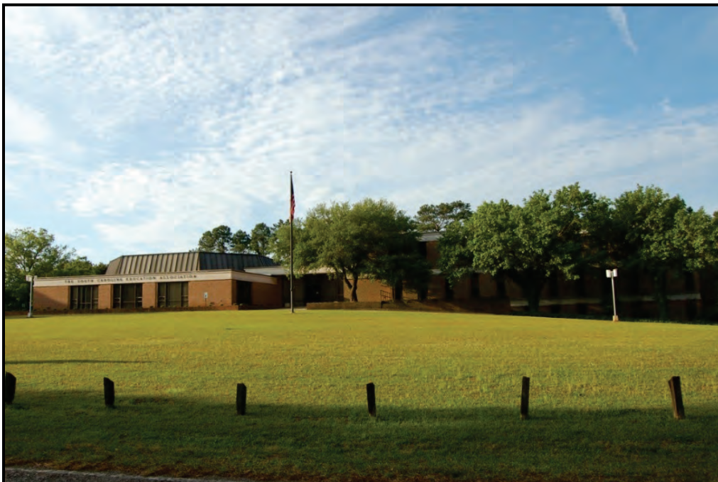
Figure 5.49: Resource 106-0880 (421 Zimalcrest Drive) – View of the facade, facing northeast.
