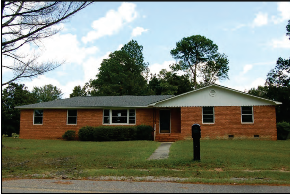
Figure 5.20: Resource 106-6394.01 (Arrowwood South Subdivision) – Representative view of property within the subdivision located at 900 Brantley Street, facing northeast.
