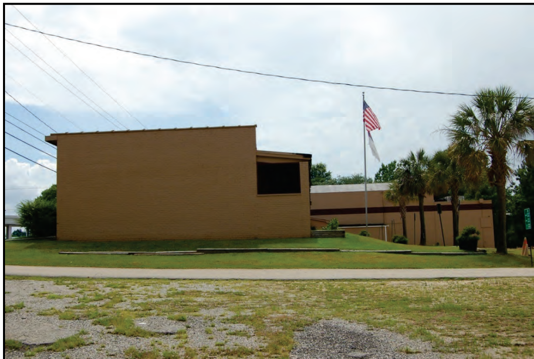
Figure 5.83: Resource 106-6407 (1311 Marley Drive) – View of the east side elevation, facing west.
