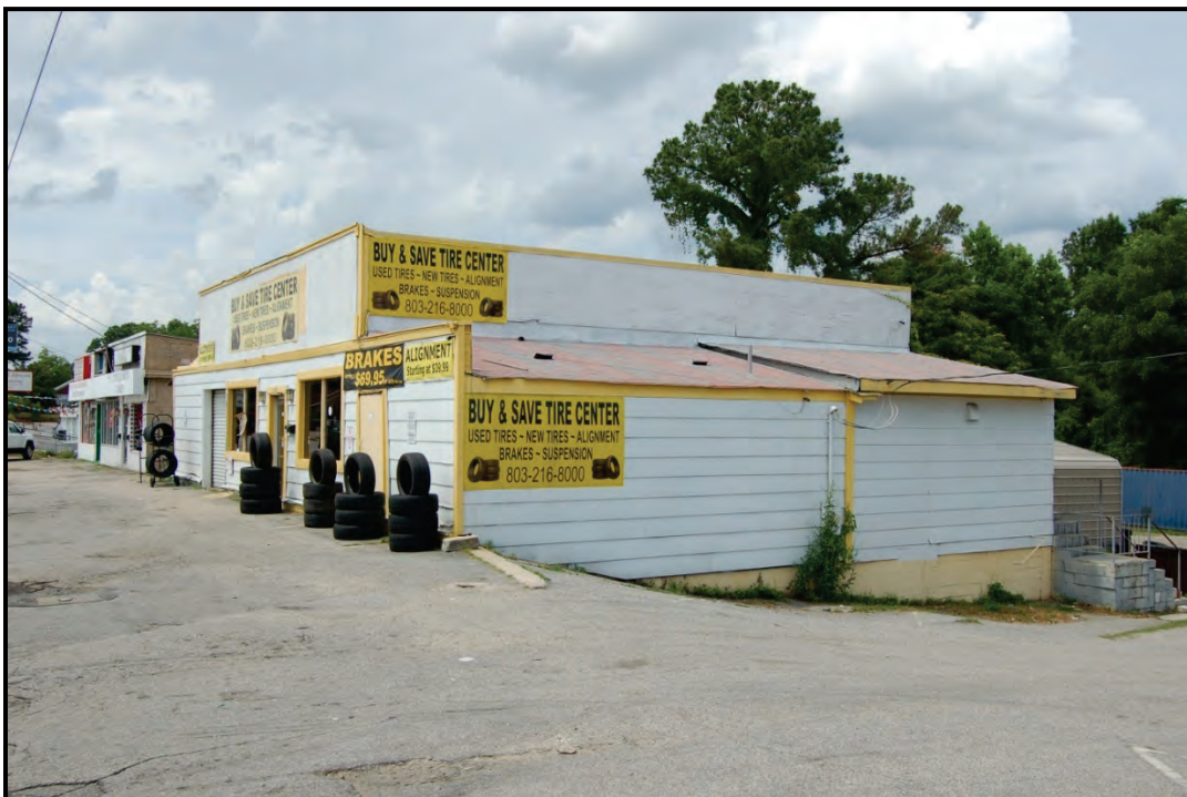
Figure 5.81: Resource 106-6406 (2420 Broad River Road) – Oblique view of the façade and south side elevation, facing northeast.
