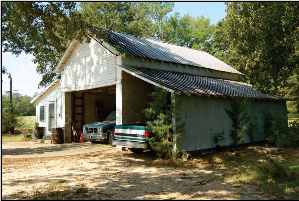
Figure 5.75: Resource 243-6467.02 (200 Roof Lowman Road) – View of outbuilding associated with the resource, facing northwest.
