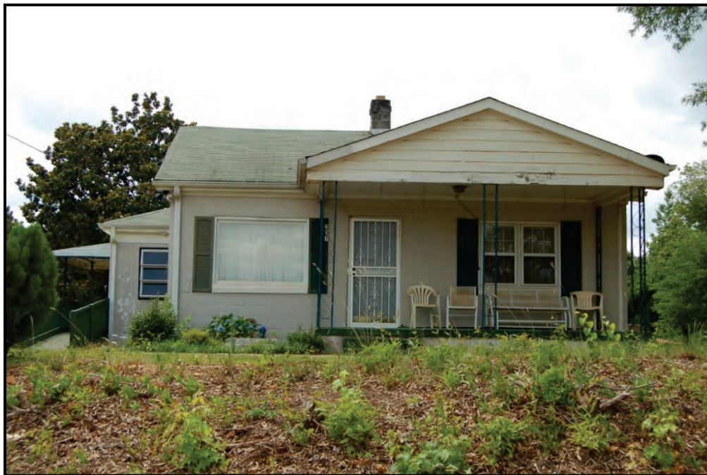
Figure 5.65: Resource 243-0885 (301 Paris Road) – View of the façade, facing south.
