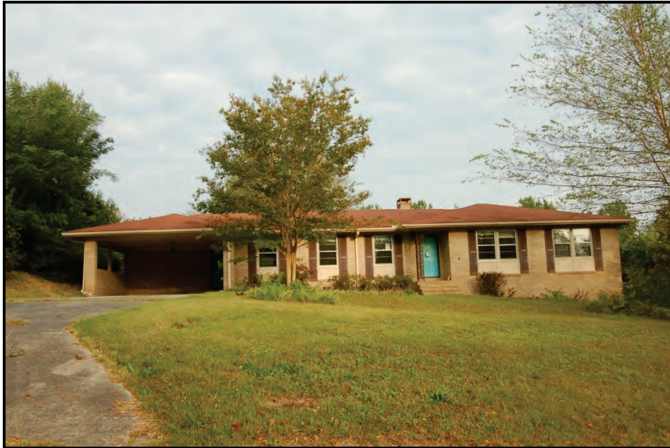
Figure 5.7: Resource 106-0878.01 (Westover Acres Subdivision) – Representative view of property within the subdivision located at 1814 Robin Crest Drive, facing southeast.
