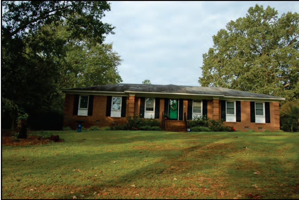
Figure 5.9: Resource 106-0878.03 (Westover Acres Subdivision) – Representative view of property within the subdivision located at 2460 Robin Crest Drive, facing west.
