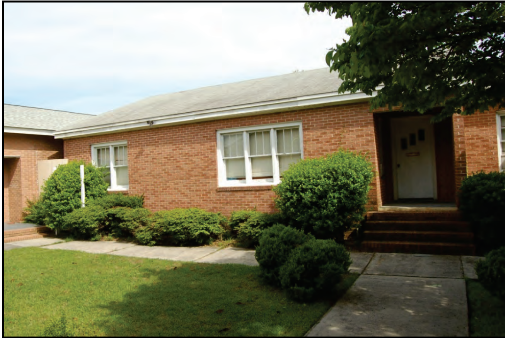
Figure 5.2: Resource 106-0877 (2500 Sunset Boulevard) - View of the façade of the original building facing north.
