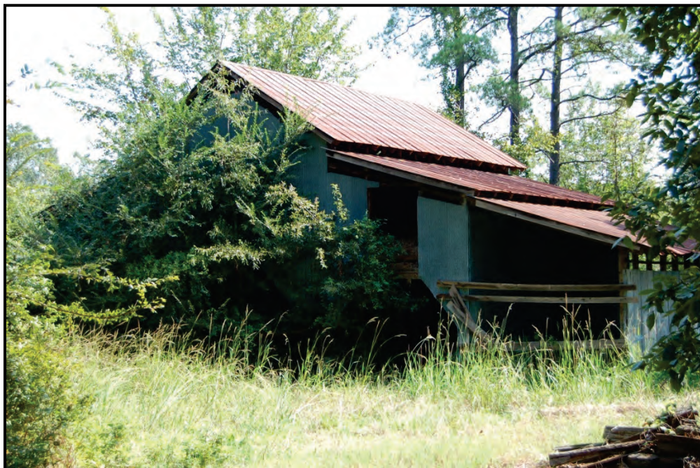
Figure 5.74: Resource 243-6467.01 (200 Roof Lowman Road) – View of barn associated with resource, facing east.
