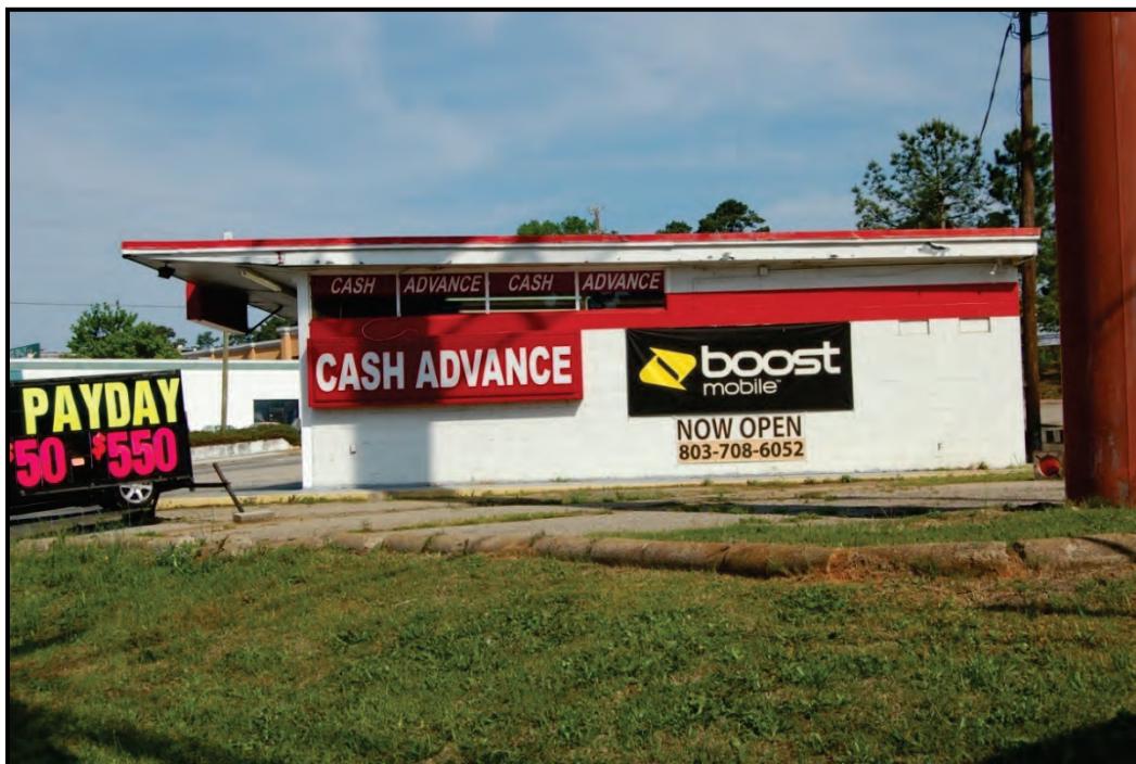
Figure 5.37: Resource 106-6396 (859 Bush River Road) – View of the east side elevation, facing northwest.
