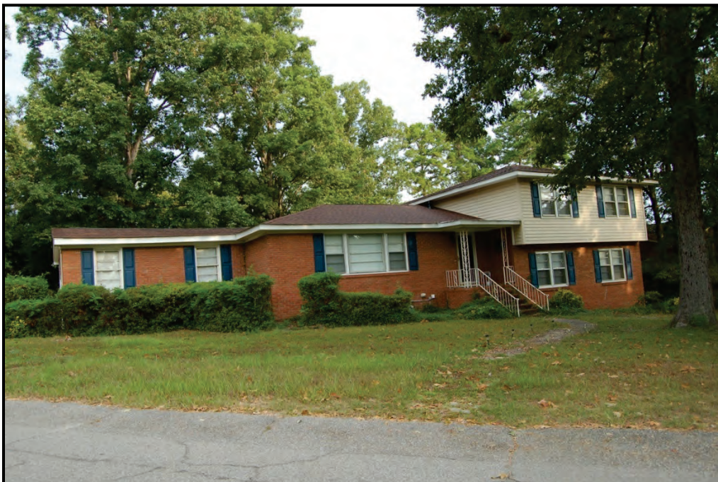
Figure 5.8: Resource 106-0878.02 (Westover Acres Subdivision) – Representative view of property within the subdivision located at 1836 Terrace View Drive, facing northwest.
