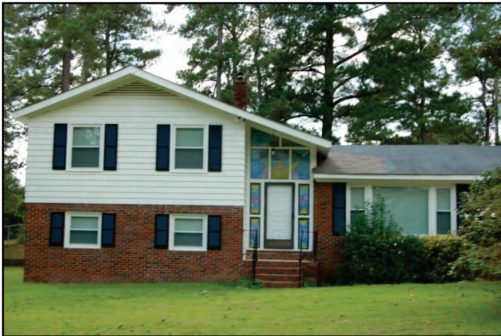
Figure 5.21: Resource 106-6394.02 (Arrowwood South Subdivision) – Representative view of property within the subdivision located at 915 Brantley Street, facing northeast.
