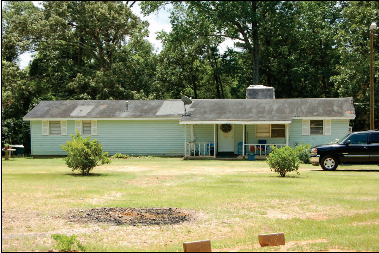
Figure 5.62: Resource 243-0882 (128 Steward Drive) – View of the west elevation, facing south.
