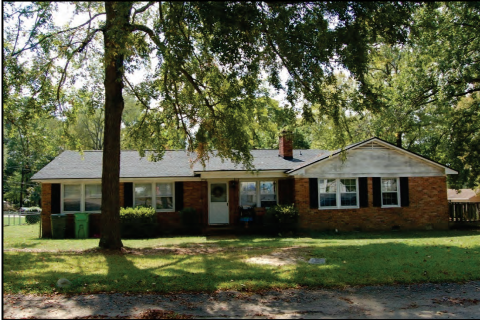
Figure 5.30: Resource 106-6392.01 (Latonea Subdivision) – Representative view of property within the subdivision located at 205 Latonea Drive, facing south.
