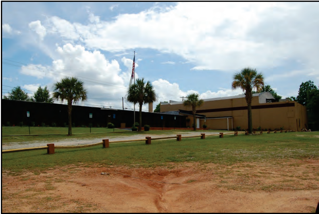
Figure 5.84: Resource 106-6407 (1311 Marley Drive) – Oblique view of the rear elevation, facing southwest.
