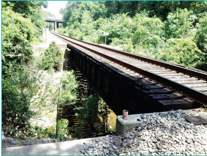
Figure 4.8. Photograph of current railroad trestle at 38RD277, facing east.
