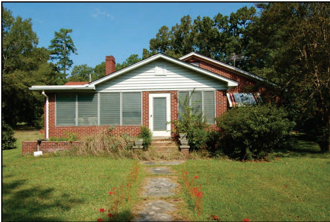
Figure 5.72: Resource 243-6467 (200 Roof Lowman Road) – View of the façade, facing north.
