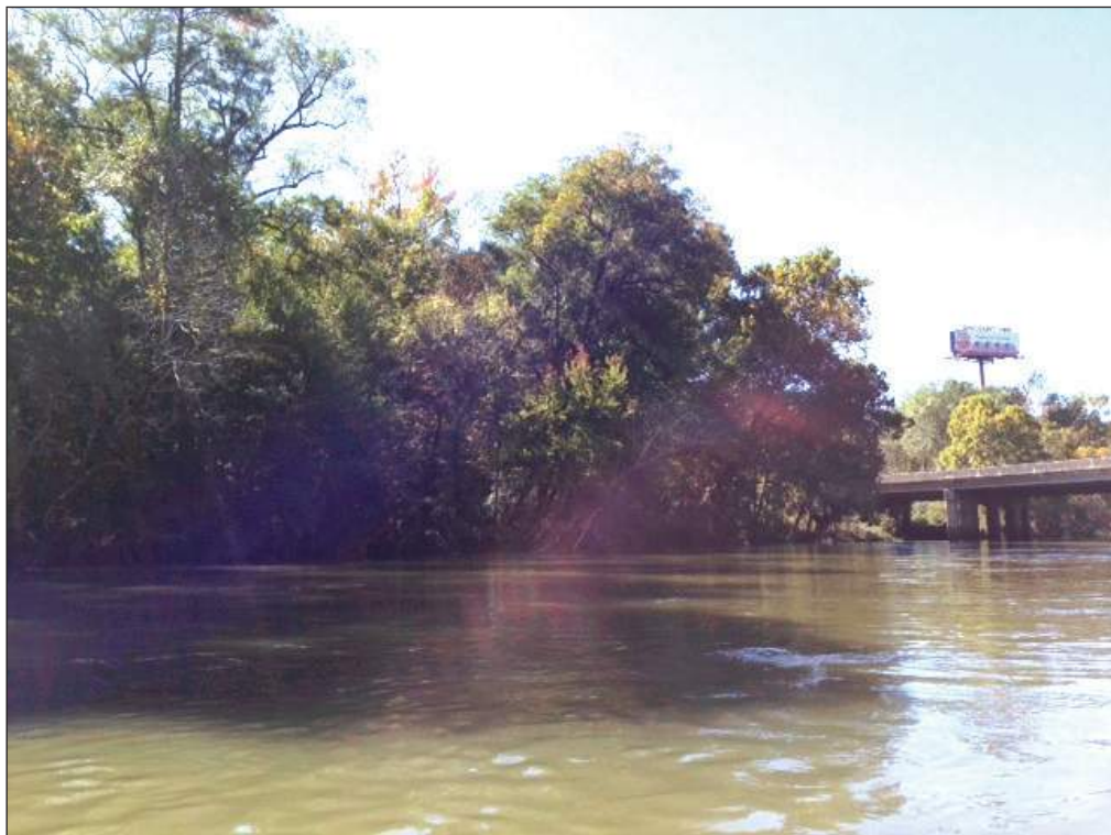
Photograph 4. View of the northern side of the Saluda River at the Interstate 20 bridge crossing.
