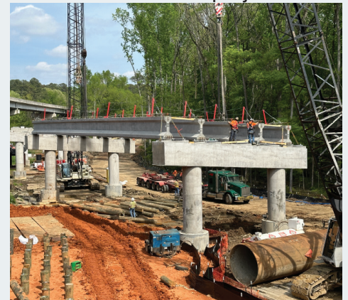
Girders being set near Saluda River near I-26 westbound.
