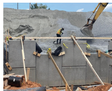
Phase 2 MSE wall construction.
