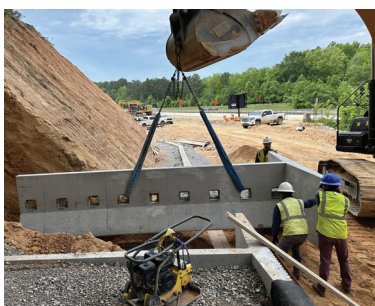
Phase 1 precast retaining wall construction.
