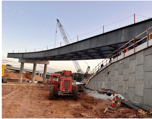
Steel girders set.
