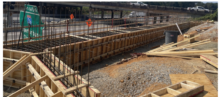
Approximately 142 tons of reinforcing steel have been installed.
