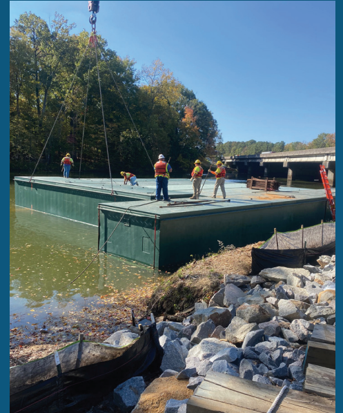
Saluda River bridge barge under I-26 westbound
