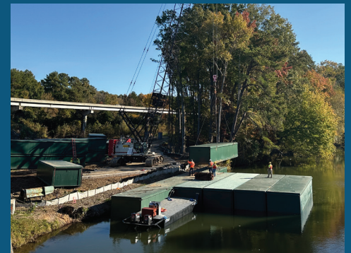
Saluda River bridge barge under I-26 westbound
