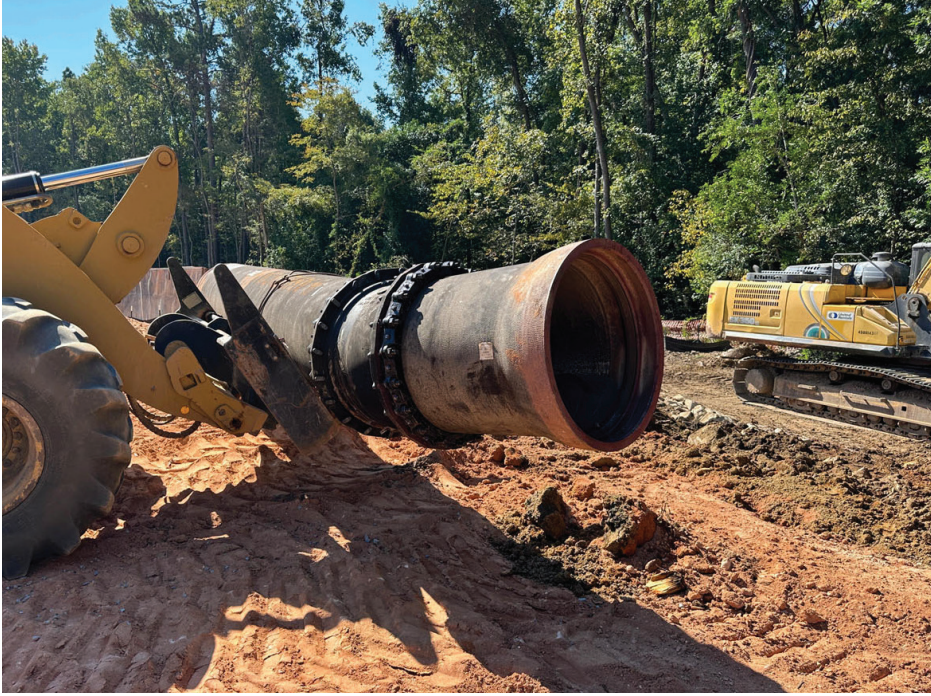
Left: Thirty-inch force main pipe fitting with a 45-degree bend. This is being installed in the area between eastbound I-126 and Saluda River. This is part of City of Columbia's sewer line relocation to allow construction of Phase 1. Right: Drilled shaft work is underway to lay the foundations for a new bridge at the Colonial Life Boulevard Interchange at I-126.
