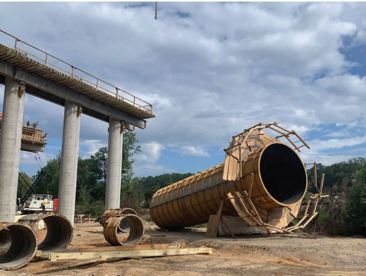
Steel form used to create concrete columns.
