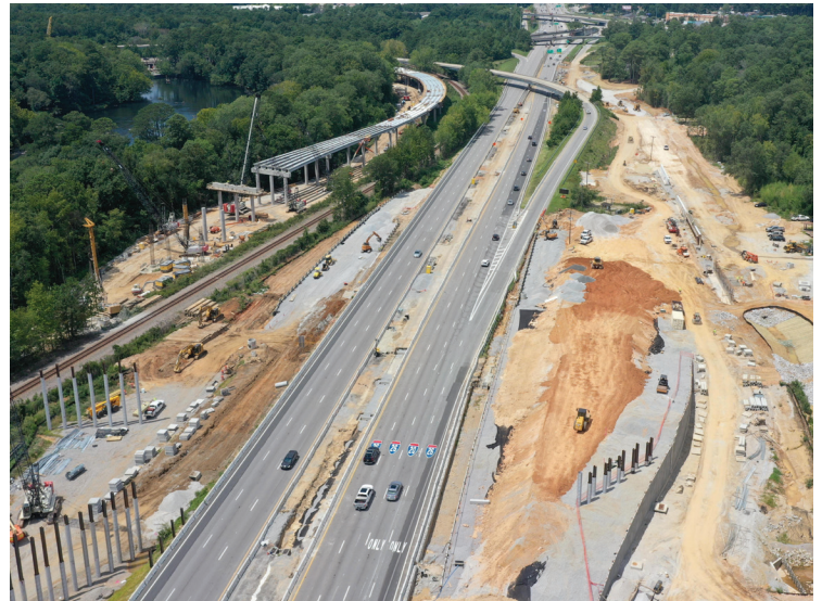
Three new bridges under construction along I-126.
