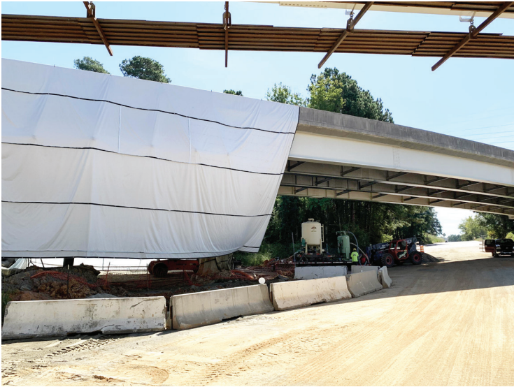
Bridge along Colonial Life Boulevard being painted.
