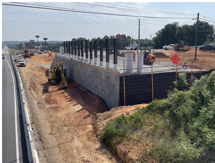
A retaining wall being constructed along I-20 near Broad River Road.
