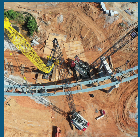
Steel girders being supported by three cranes.
