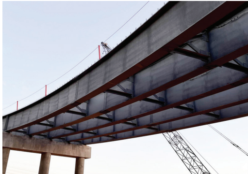
Steel girders for Ramp from Colonial Life Blvd to I-126 westbound.
