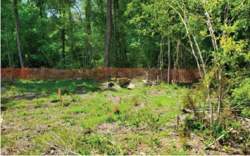
Tributary 39. Photo courtesy of Widlands Engineering, Inc.
